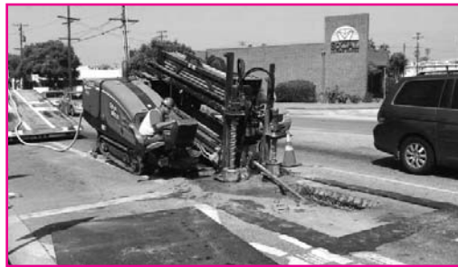
Directional drilling rig installing conduit for utility relocation
