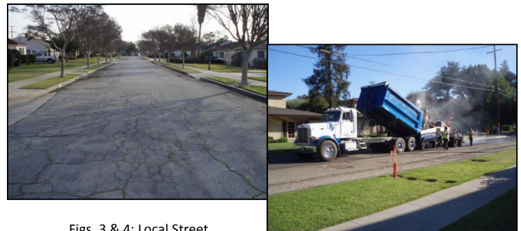
Figs. 3 & 4: Local Street Rehabilitation
